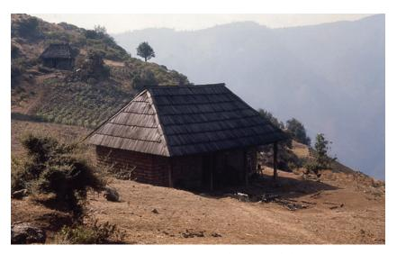
FIGURE 1.12. A typical house in Patalcal: walls of adobe, roof of wood shingles. The porch and patio in front of the house are the principal work areas. Photo by the author.
