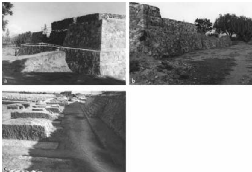
9.5. North, south, and west walls of Mound 195
