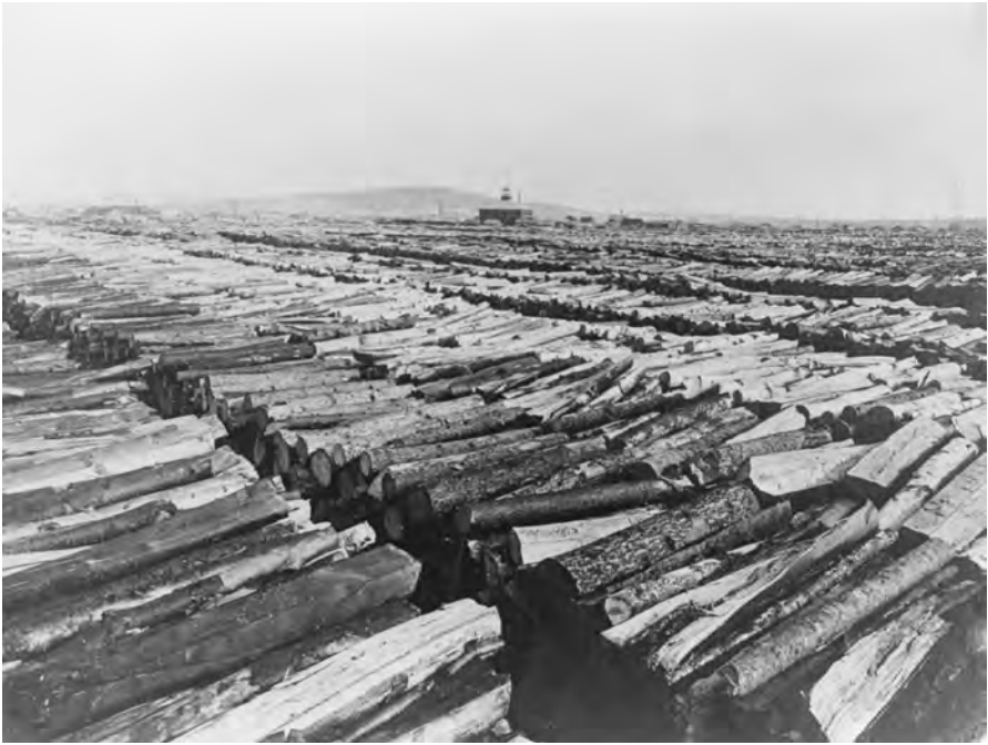
Wood yard at Tanana River Railway, ca. 1905–1910. Cole coll. 76-38-20, University of Alaska Fairbanks, Alaska and Polar Regions Archives. The railroad burned wood in its locomotives, used it for railroad ties, and delivered it to mining sites. Added to forest fires, the use of wood for mining, steamboats, railroads, heating, and power generation stripped many hills and valleys of trees.
