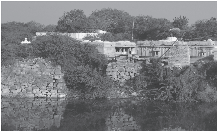
Figure 3.4. Gabbur water management feature known as Elu Bavi (“Seven Well”), west side. Author photograph.
