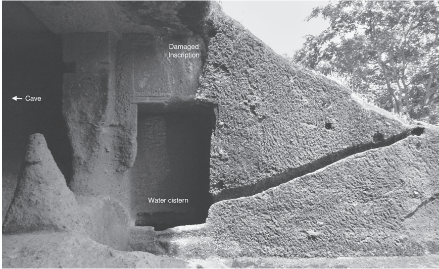
Figure 3.1. Example of a water cistern attached to a monastic cave at Kanheri, western India. Water from the surface is directed to the cistern through a channel dug into the rock of the hill (the niche above the cistern is about 1.7 m high). Author photograph.
